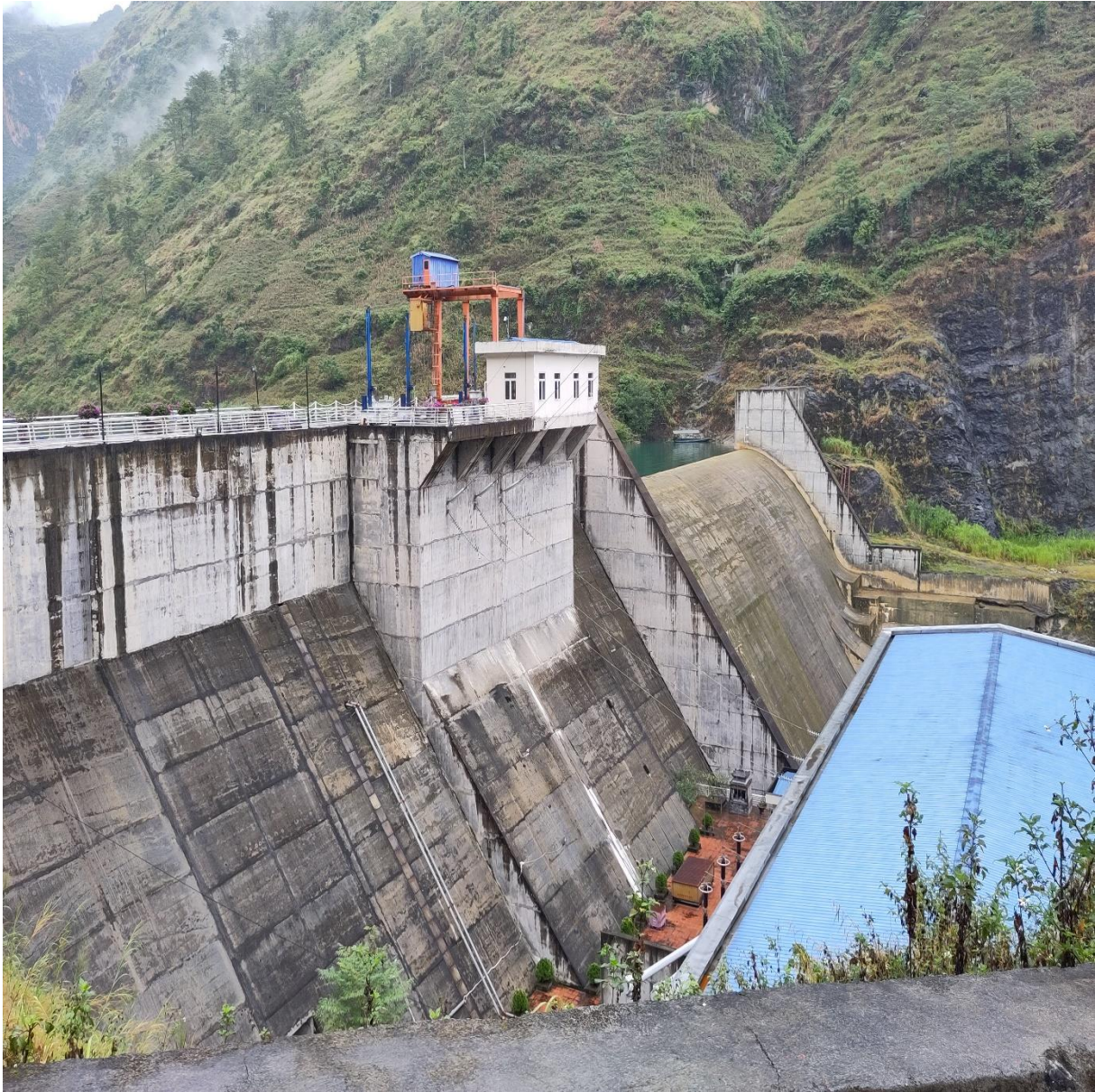
Picture 24: Weir near Ha Giang
